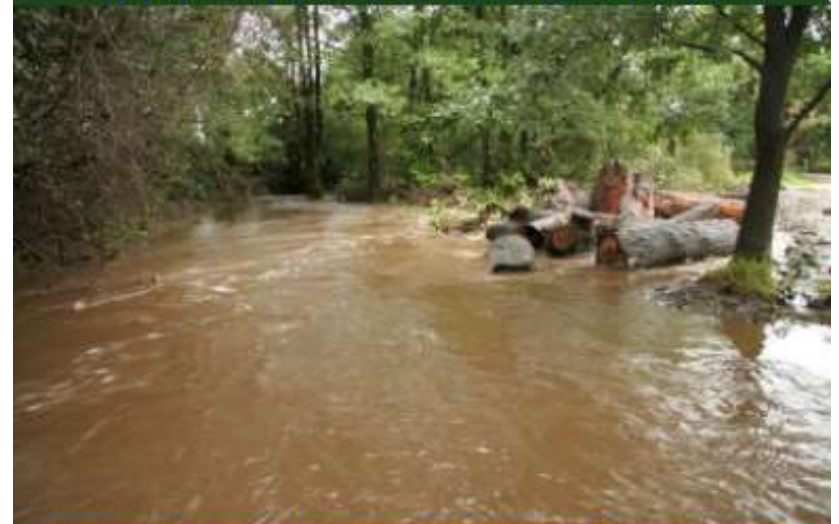
September 2009. It works! Just two weeks after the ELJ had been completed, a late summer storm resulted in spate conditions. The position of the ELJ re-activated an old channel. It is estimated that, at the peak, a third
