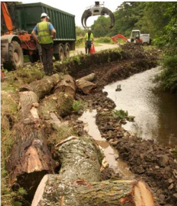
August 2009. The gabion baskets were removed and replaced with living, sprouting willow trunks.
