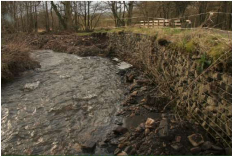
View of the collapsing gabions in 2008
