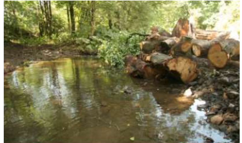
View of the completed ELJ and the entrance to an old side channel.
